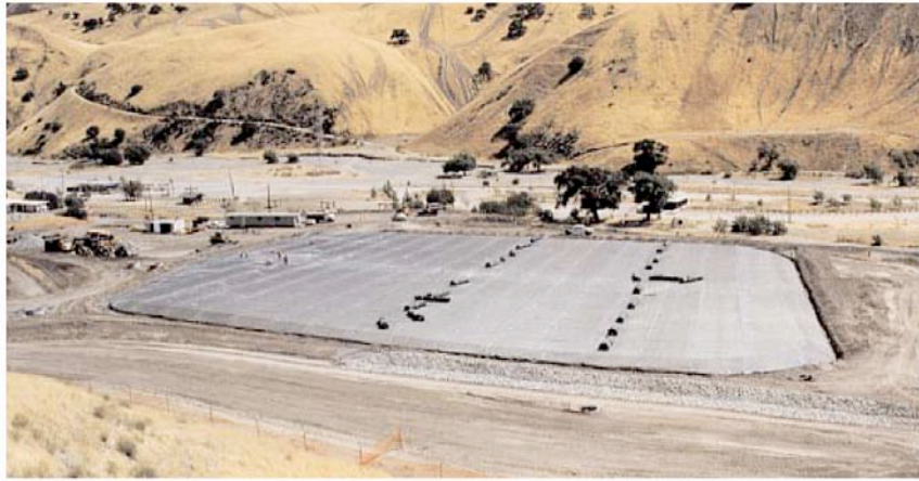
Pit 6 Landfill liner during installation; view looking south (July 1997).
