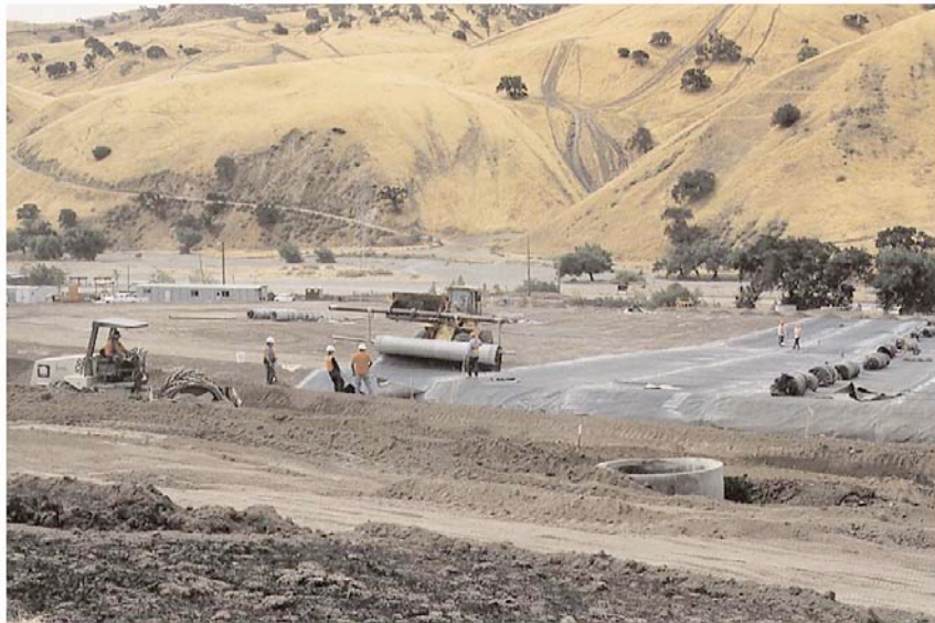
Installing the HDPE/geosynthetic clay liner (July 1997).
